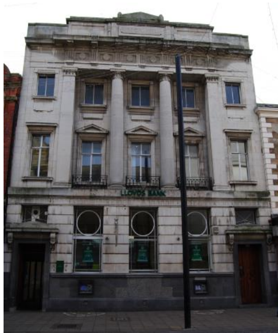
Lloyds Bank (grade II listed)
