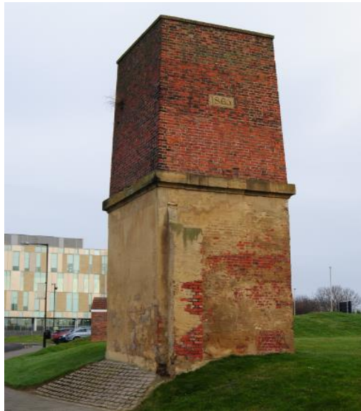
Chimney, former Cookson Glassworks, Harton Staithes
