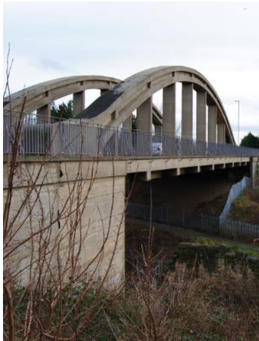
Bridge, River Drive
