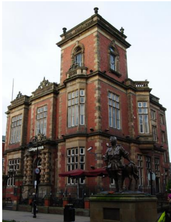
The former Marine School (grade II listed)
