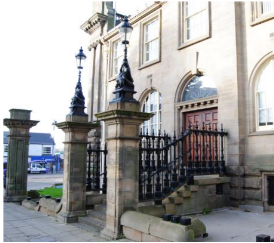
Railings and Piers to the Municipal Buildings (grade II listed)
