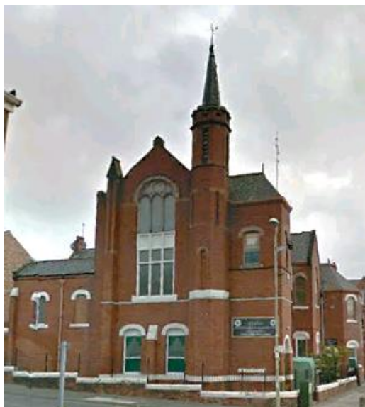
Baitul Malmur James-e-Masjid and Islamic Centre
