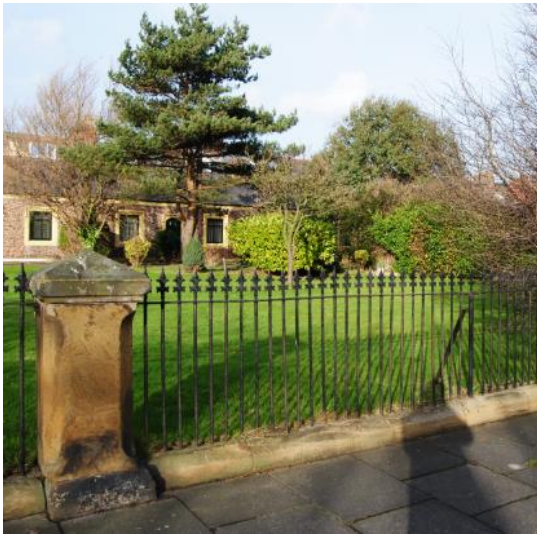
Boundary Wall to No's 1 to 21, fronting road (grade II listed)
